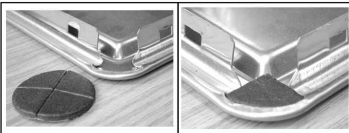
Remove the protective back from the main seal and stick to the underside of sink.
